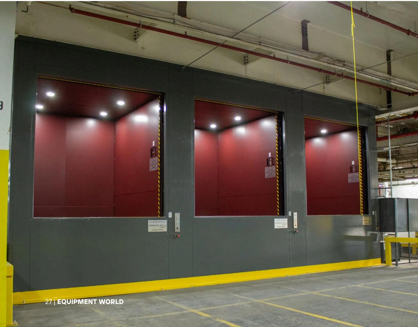
Unlike passenger elevators, material lifts are specifically engineered for the efficient movement of goods and products, making them the most cost-effective and straightforward solution for lifting loads.
