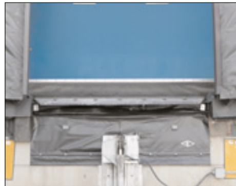
Pit sealed with PitMaster.
